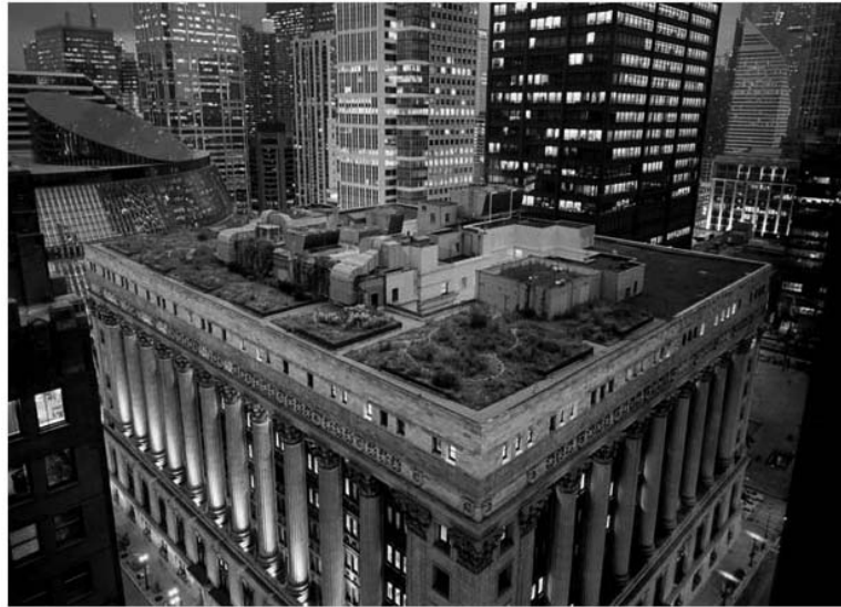
Up on the Roof
